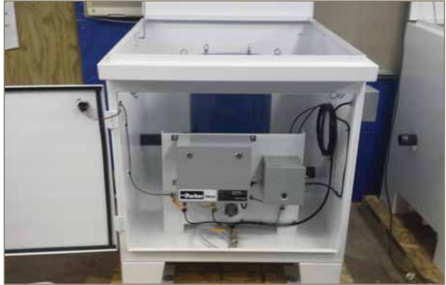
AFS Diesel Filtration Skid Enclosure with Parker Velcon IPM-230.
