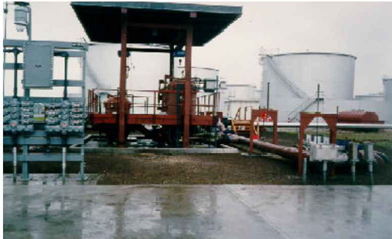
The JFK Airport fuel farm underwent reconstruction to achieve greater efficiency.
