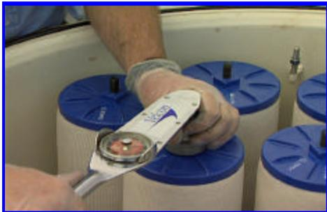
Model numbers on the elements must agree with records. Check that they meet any applicable standards, e.g., API 1581 or IP Monitor Spec.).
