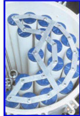
Check the condition of the spider plates. They should be secured properly and in good condition.
