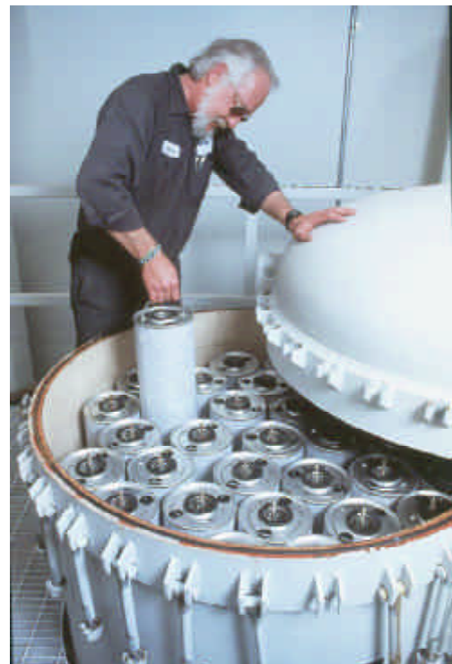
Installing clay cartridges
